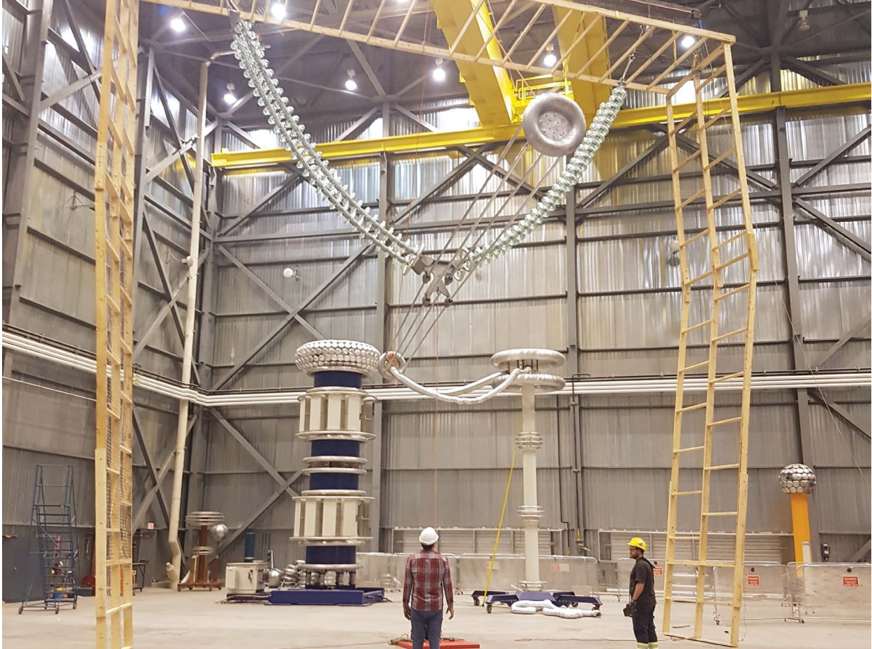
Visual corona and RIV testing on double v-string transmission line assembly.
